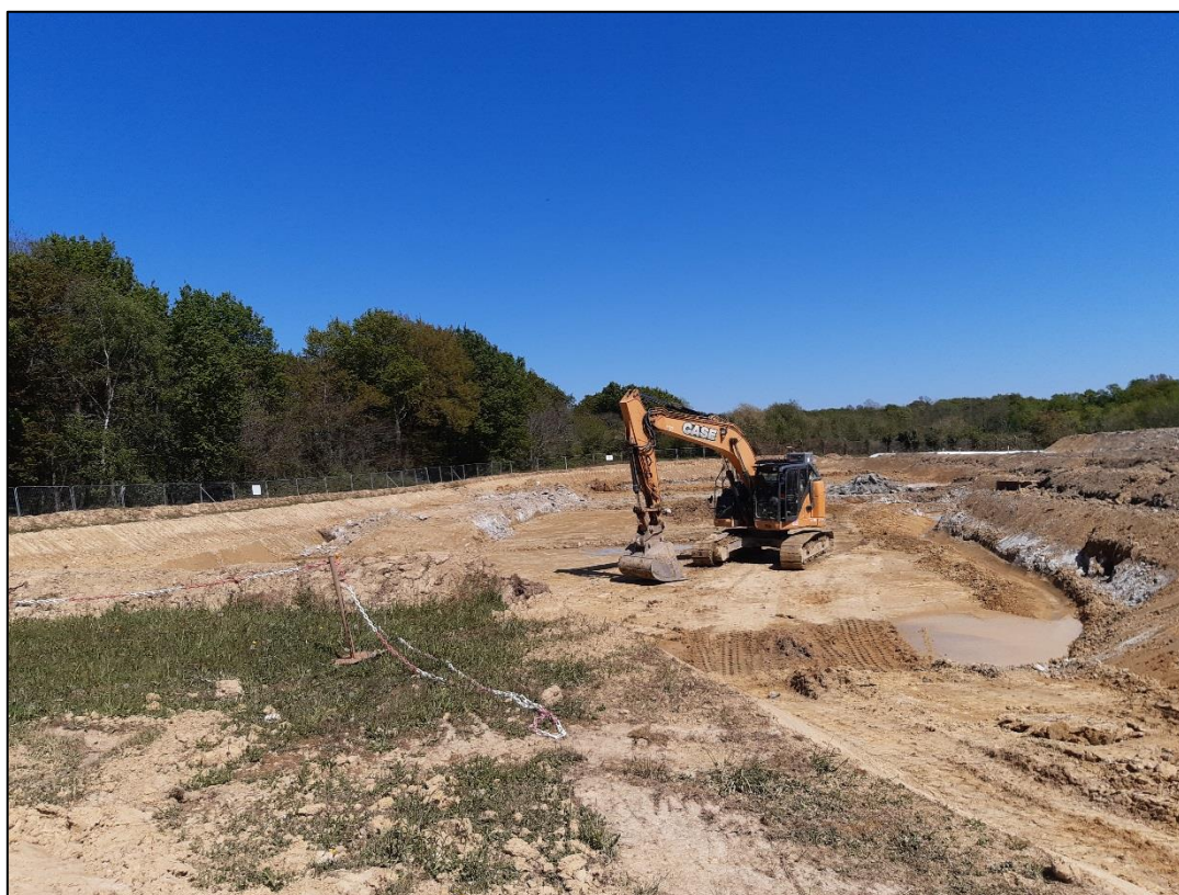
Figure 6 : Excavation d'un borbier (BURGEAP)
